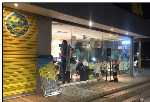
Fig. 47 - The Programo tu Futuro building is designed to inspire the local community
