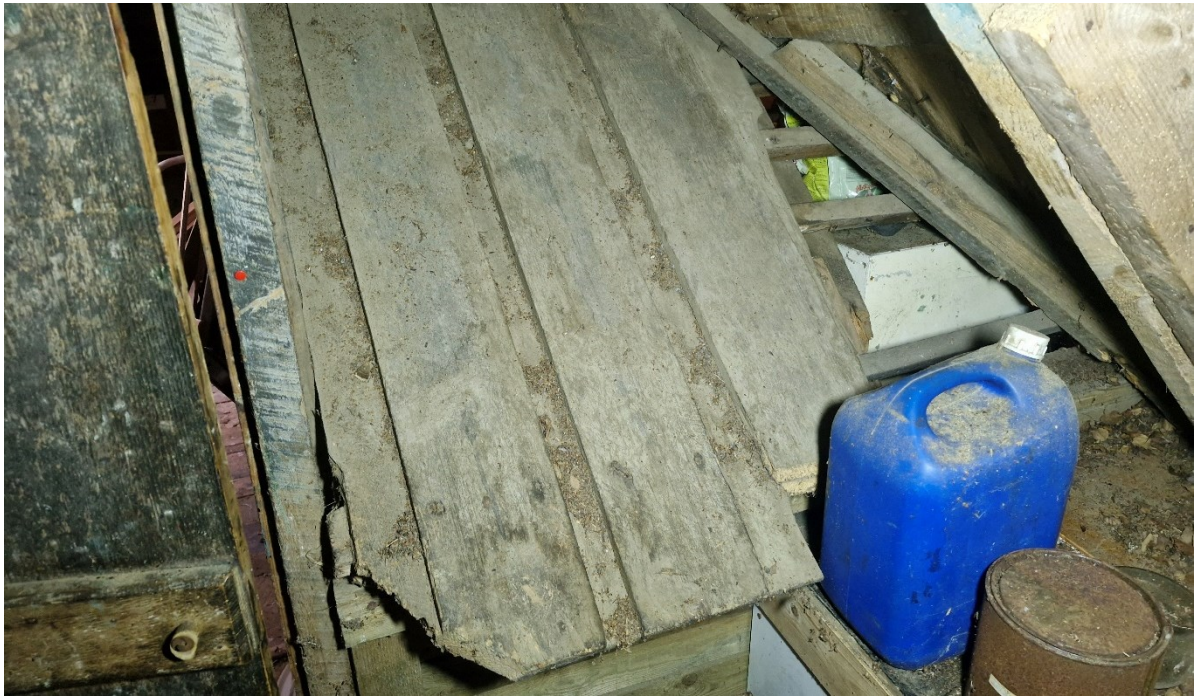
Preserved section of historic planked roof, inside the 1853 Finzean Bucket Mill, Aberdeenshire. Roofing shingles are not the only pattern of wooden roofing found in Scotland.
