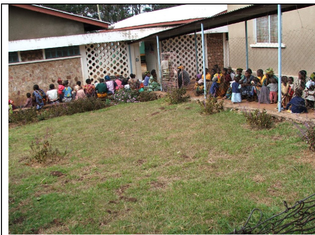
The waiting room for the Primary Care Unit at Murgwanza Hospital
