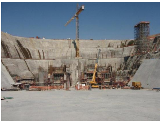
Construction of the two inlet tunnels on the upper Bedford dam.
