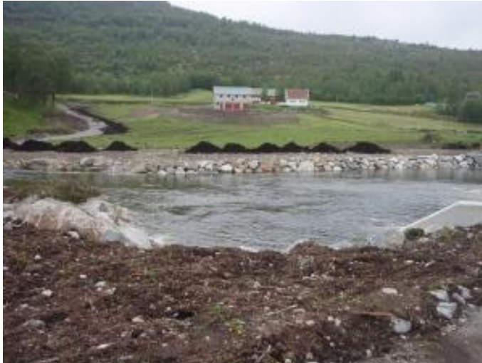
Landscaping work in progress around Dalavatn dam.
