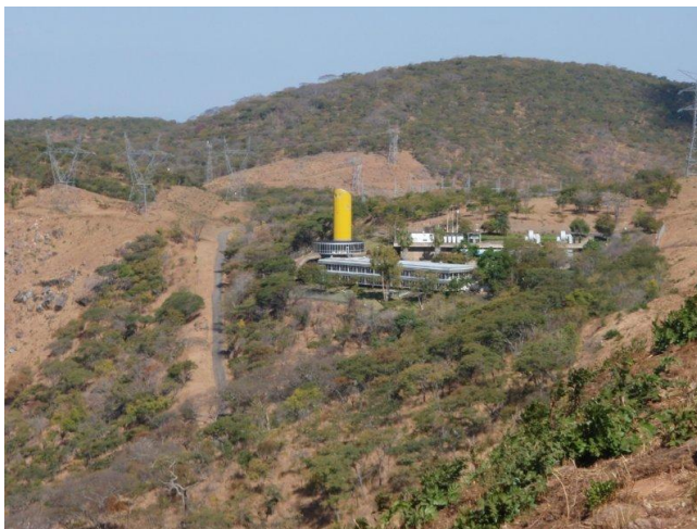
View of the station.
