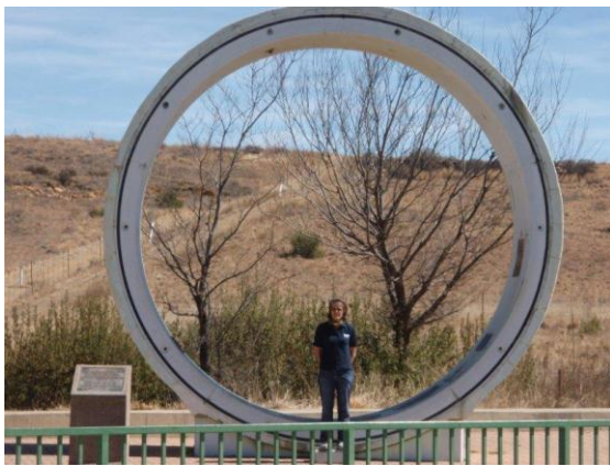
Standing inside a typical section of the 5m diameter Lesotho transfer pipeline.
