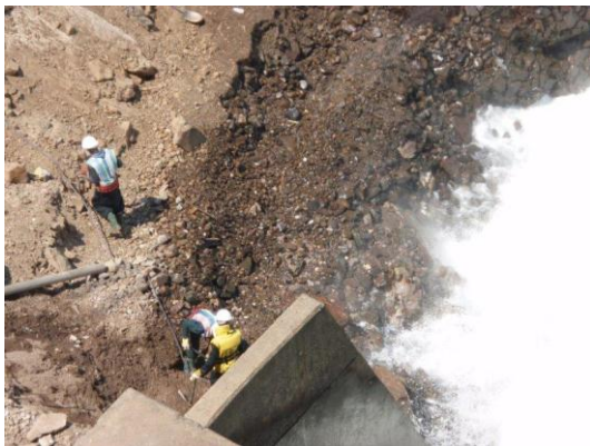
Workers replacing gabion baskets – an ongoing battle.
