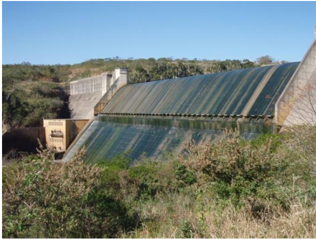
Nahoon dam wall, with the water levels just overtopping at the time of the visit.
