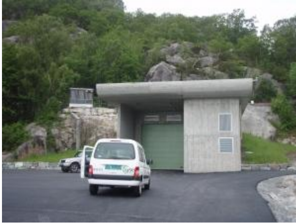
The only visible bit of the underground Jossang hydropower plant.
