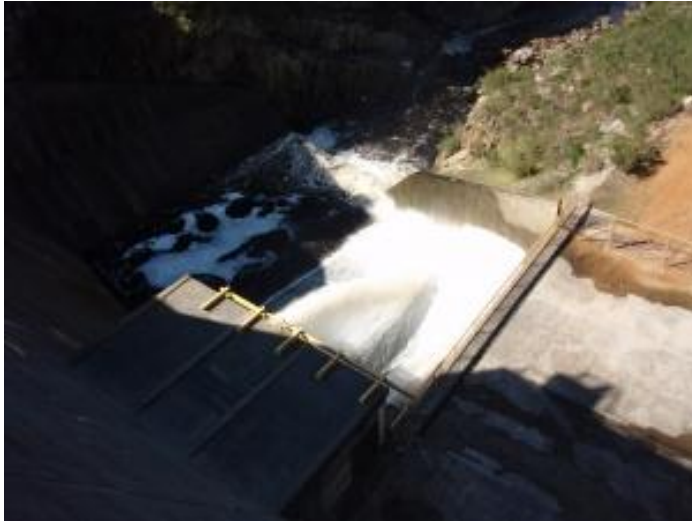
Compensation spill from Koegelberg dam - no turbine.
