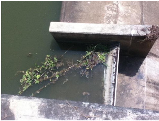
The flap gate on the side, catching weed.
