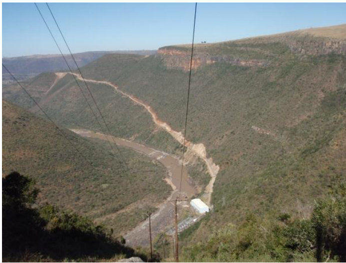
Looking down towards the Hydropower Plant – note the incredible access track.
