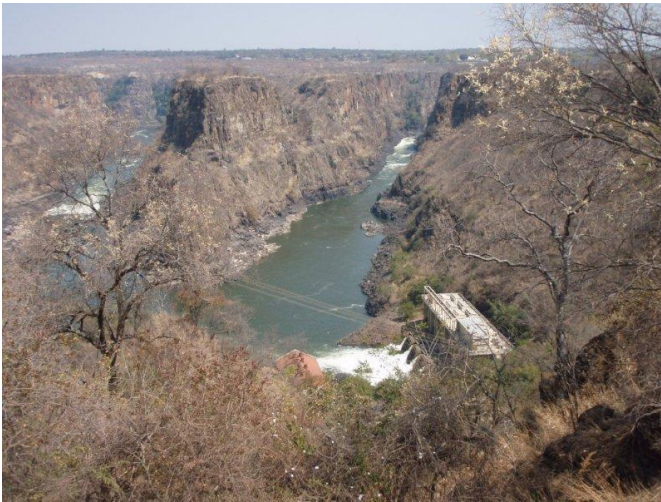
View looking down to the three hydro stations.
