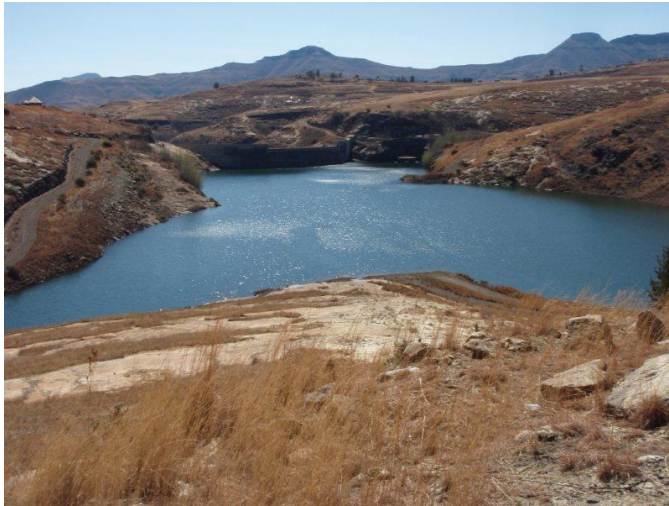
The Muela dam, showing the dam wall and intake to the gravity tunnel to South Africa.
