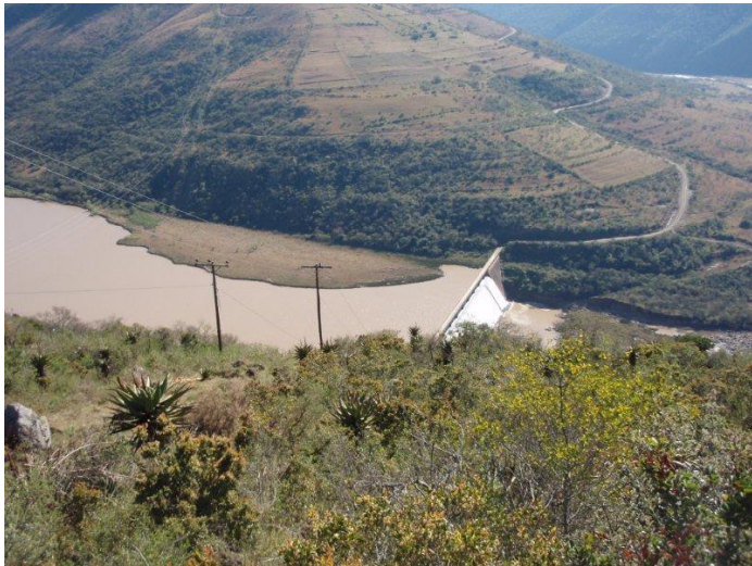
Looking down towards Mbashe buffer dam, with the silt island clearly visible.
