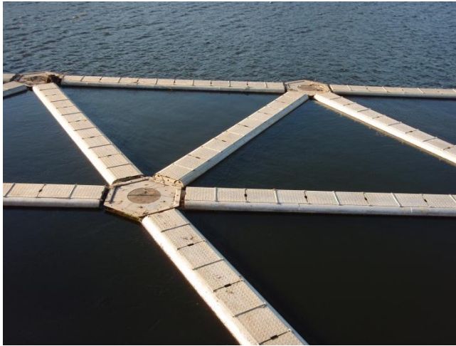
Booms installed recently at water inlet, to minimise hyacinth blocking the screens.
