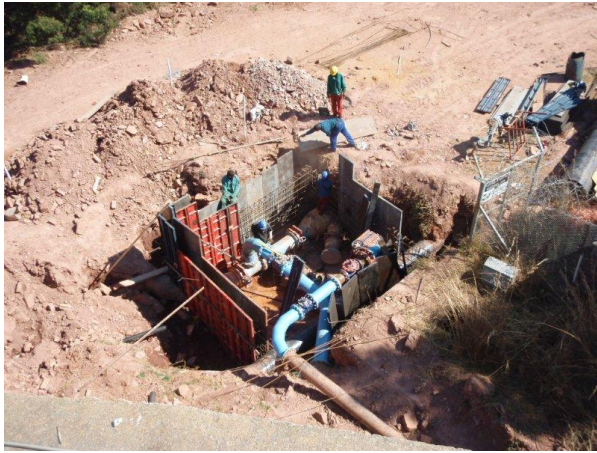
The modification to the inlet pipes is nearly complete.
