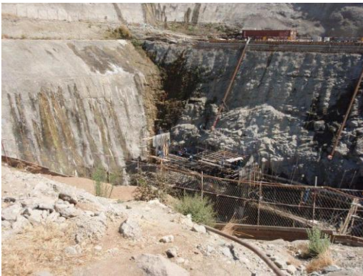
Coffer dam with works on inlet to the new turbines 5 and 6.
