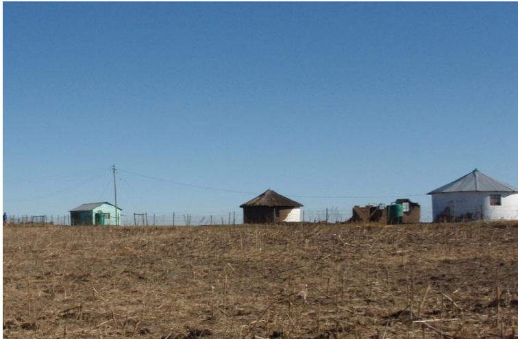
Power lines connecting rural huts.
