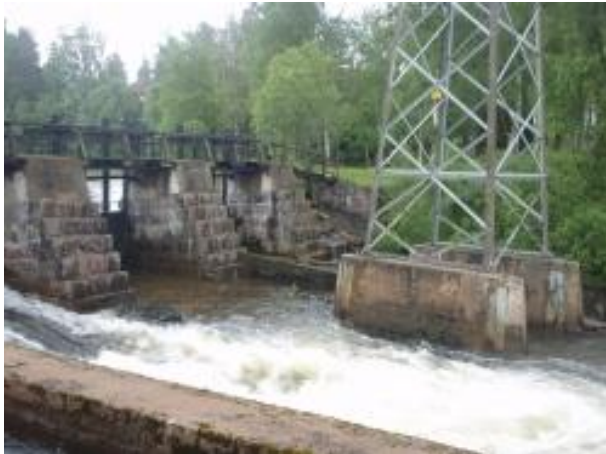
Power pylon located in the river bed below the dam wall.
