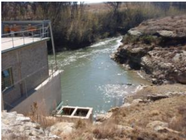
The station and location of tailrace.
