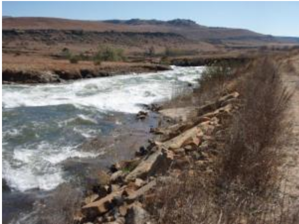
Bank reinforcement on the side of the river-side of the canal.
