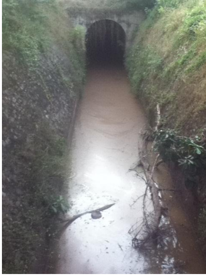
Tailrace exits into a canal, and then into the Pangani river.
