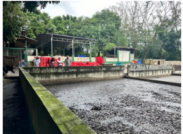
Above: Greenland chicken processing plant, Lipa City; the waste slurry pits are treated with an EM solution - there is no smell. The slurry is then fed into nearby worm windrows, where the worms turn the waste into nutrient-rich vermicompost.
