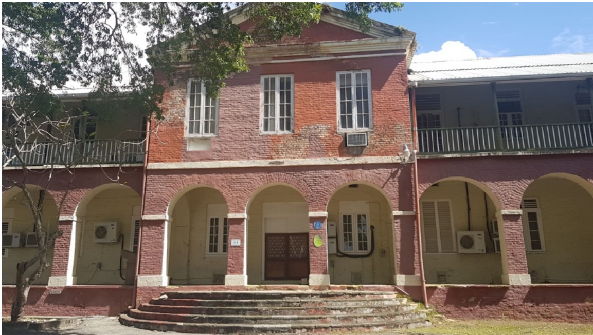
Figure 24 - Barbados (St. Ann's) Garrison, south of Bridge Town
