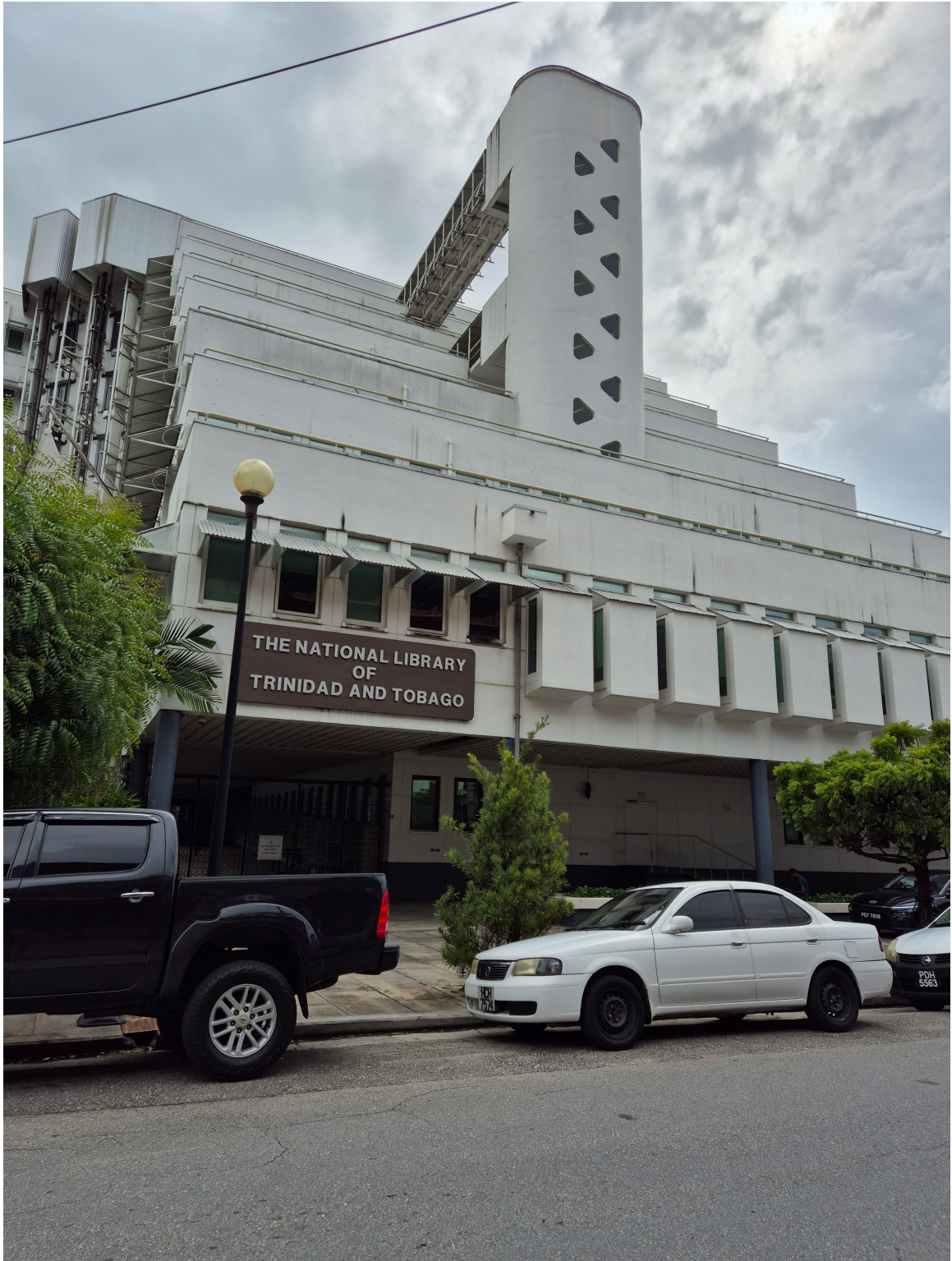
Figure 17 - National Library of Trinidad and Tobago, Port of Spain
