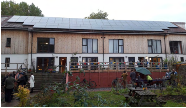
Fishponds Rd- BCLT First Project
