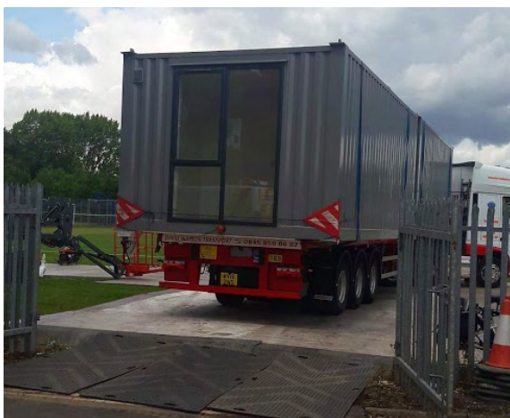
The first units arriving on site.
