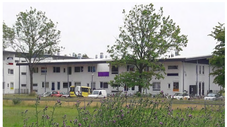
One of the Startblok blocks of 565 studios
