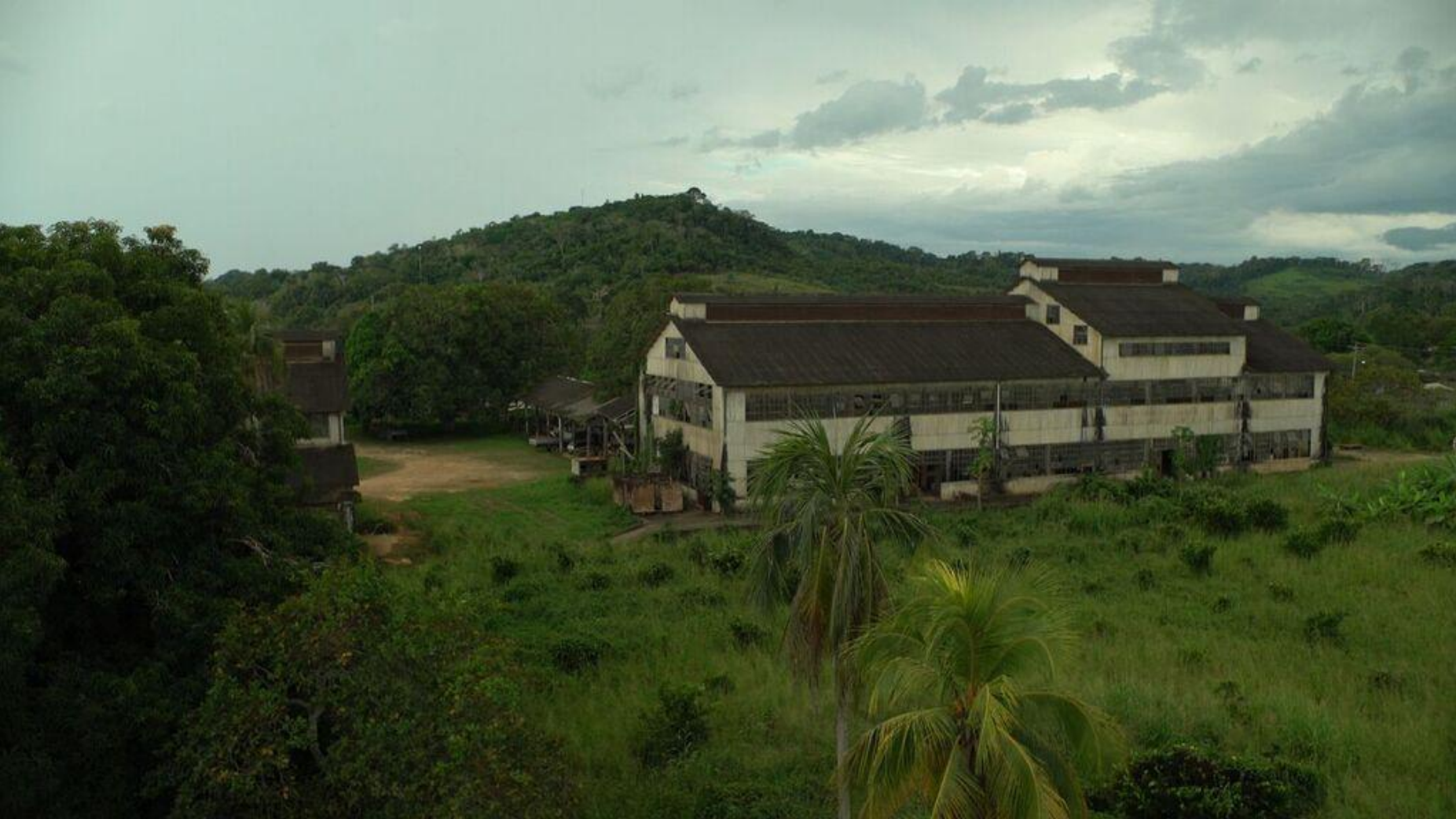
The old rubber processing factory at the heart of Fordlandia
