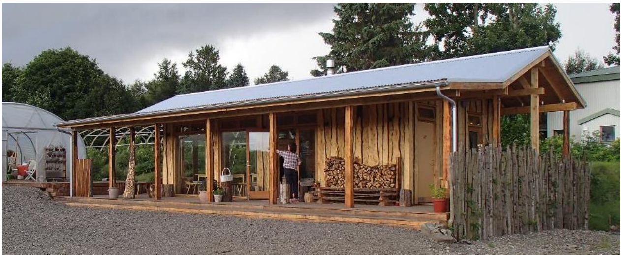
The Aspen Building, Vallanes Farm, eastern Iceland
